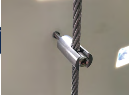
Figure 4 – Créa Diffusion had to come up with a way to coordinate the square and vertical holes so that the rails weren't visible from the interior, which it did by hanging the sheets on vertical stainless steel cables.
