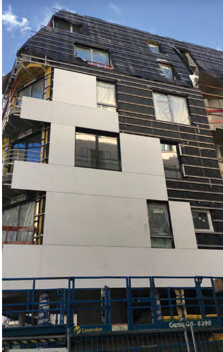
Figure 3 – One major challenge was to fix the solid surface to the rails of the aluminum structure, which had to be plumbed perfect and true to the concrete wall made by the general contractor to avoid problems.
